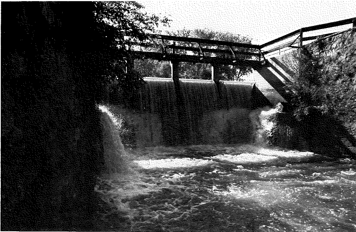
Swan Creek spillway in Lambertville
